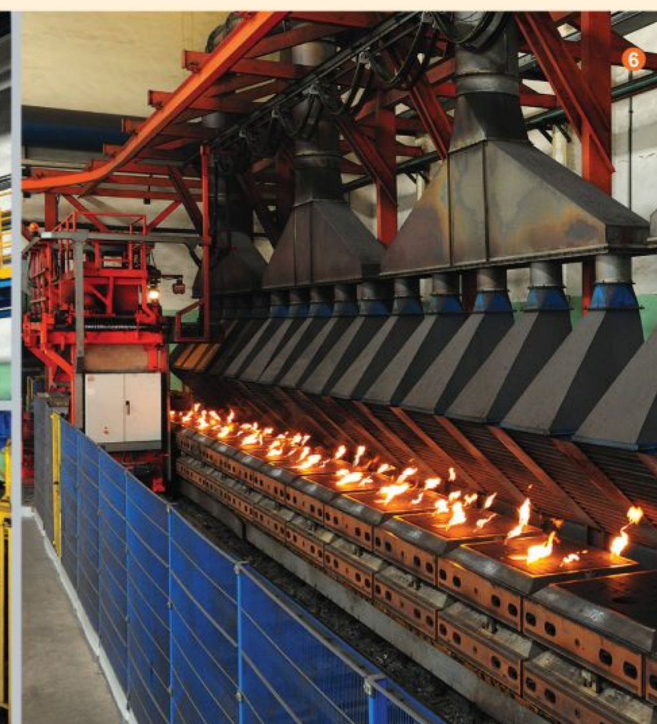
5. 德国HWS（霍氏）公司生产的静压自动造型线造型主机 The host of automatic static pressure modeling production line produced by Germany HWS (Hough) Company
